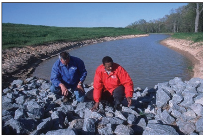
Scientists inspecting a completed tailwater recovery pond and rock rip-rap in Lonoke County, Arkansas; Natural Resources Conservation Service, USDA
