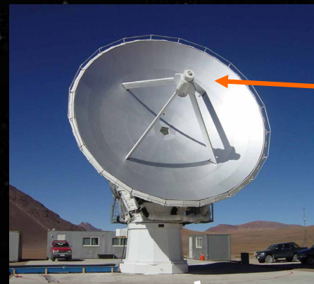
Holography Receiver at top of secondary
