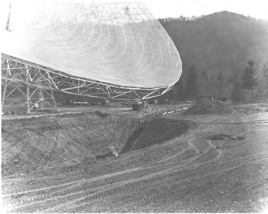
Digging the ditch to extend the southern declination limit, October 1962.
