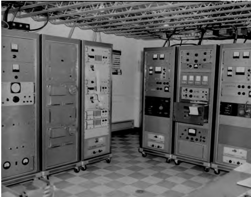
The 40 Foot Telescope and its underground Control Room in 1962.
