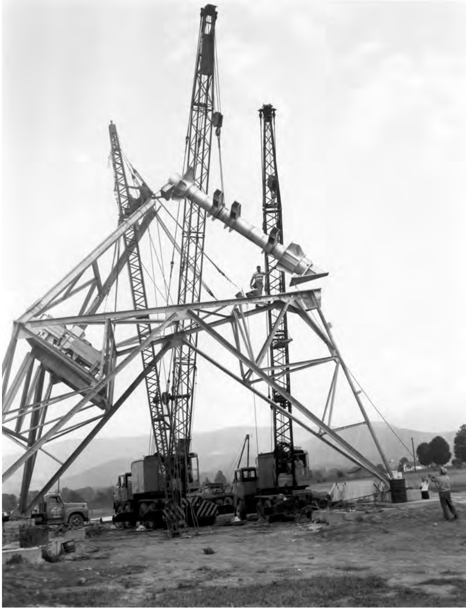
Installation of the polar shaft on the 85 Foot Tatel Telescope.
