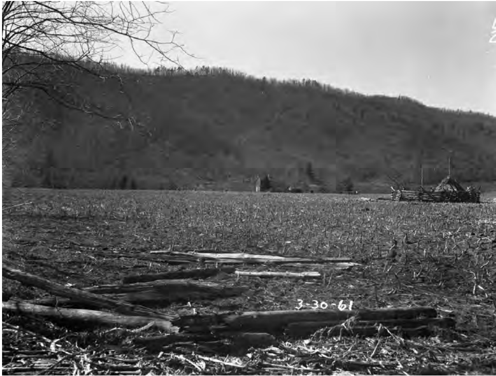
The site of the 300 Foot before the start of construction, March 30, 1961.
