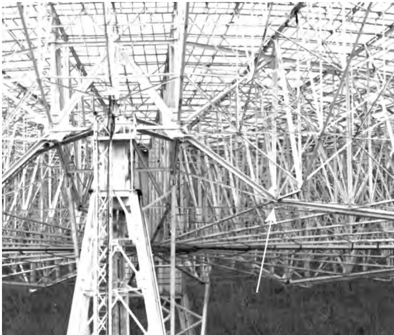
The circle (above) and arrow (below) shows the location of the gusset plate that was believed to have failed and precipitated the collapse.
