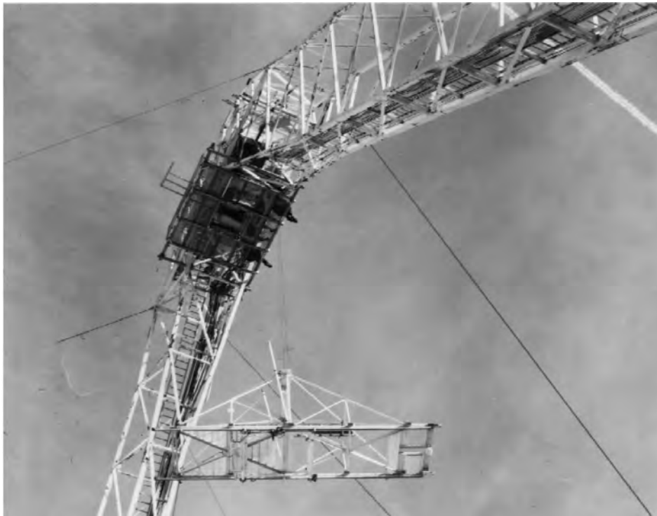
Installation of a stronger, more accurate traveling feed, October 1980.
