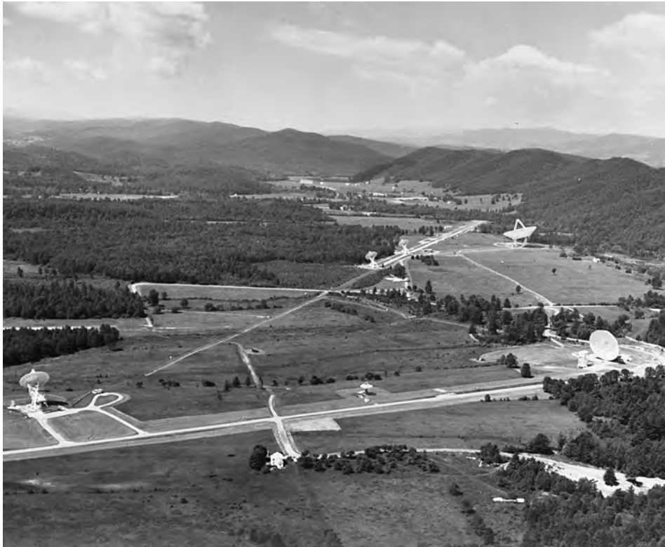
Aerial view of the Green Bank Observatory in 1980, looking south. The 300 Foot Telescope is at the top right; the 85-2 and 85-3 Telescopes to its left; the 140 Foot at middle right (in service position); the 40 Foot Telescope in the lower middle; and the 85 Foot Tatel Telescope at the lower left.
