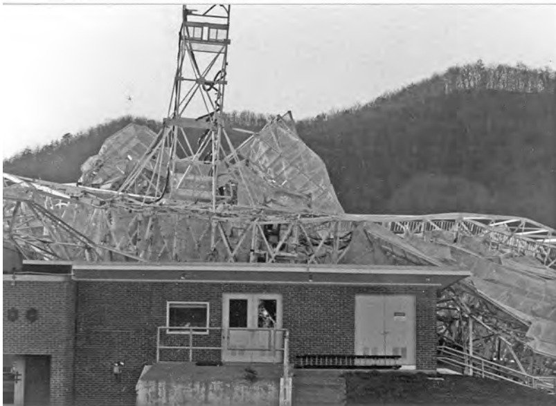
The remains of the traveling feed atop the control building. [Photo courtesy G. Liptak]
