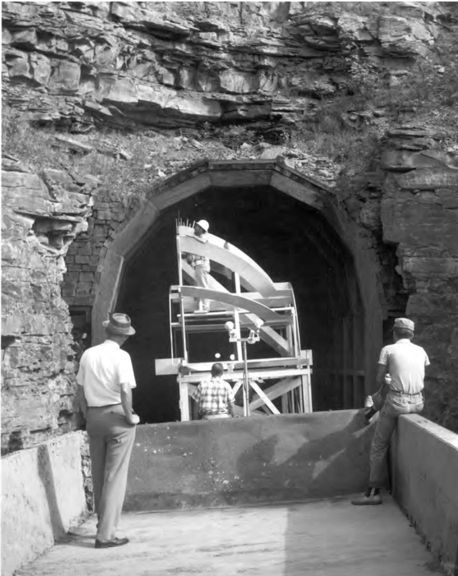
Testing a mock-up of the 17\frac{1}{2} foot spherical bearing for clearance in the rail tunnel through Droop mountain in 1961. The size of the bearing allowed for three inches of clearance.
