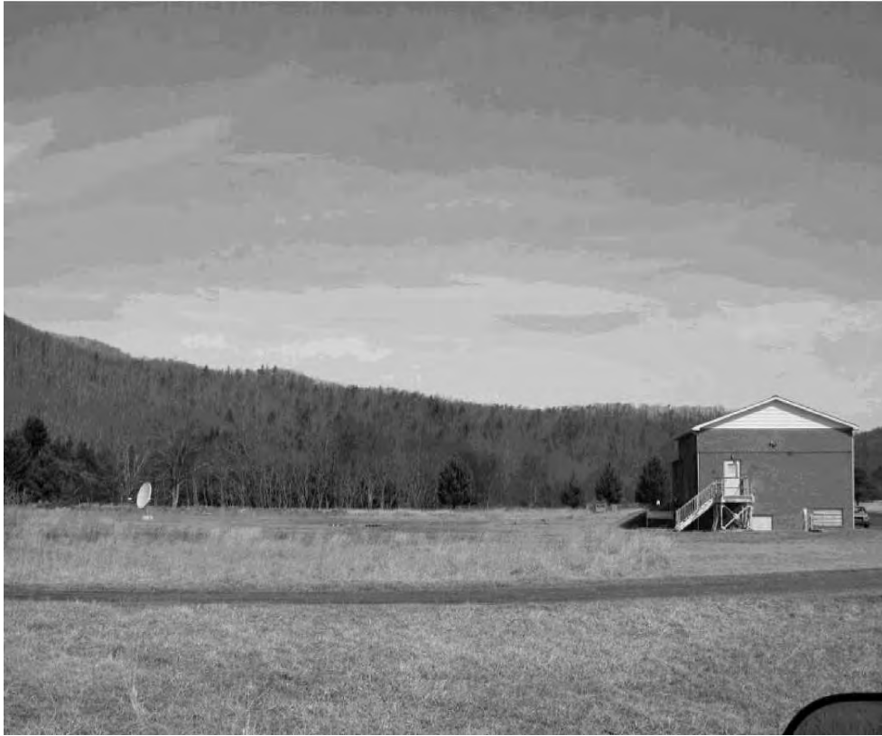
View from the South, March 2002. The Control Building, with a new roof, is now the laser ranging lab for the GBT. The 300 Foot Telescope stood in the open field to the left of the building.
