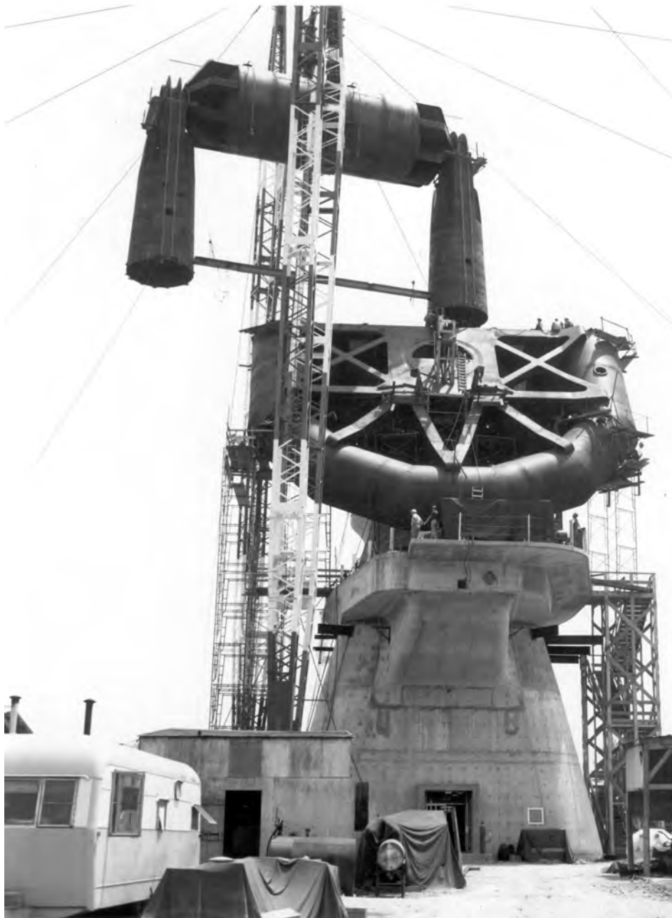
Lift of the final yoke section with a connecting ballast tank.
