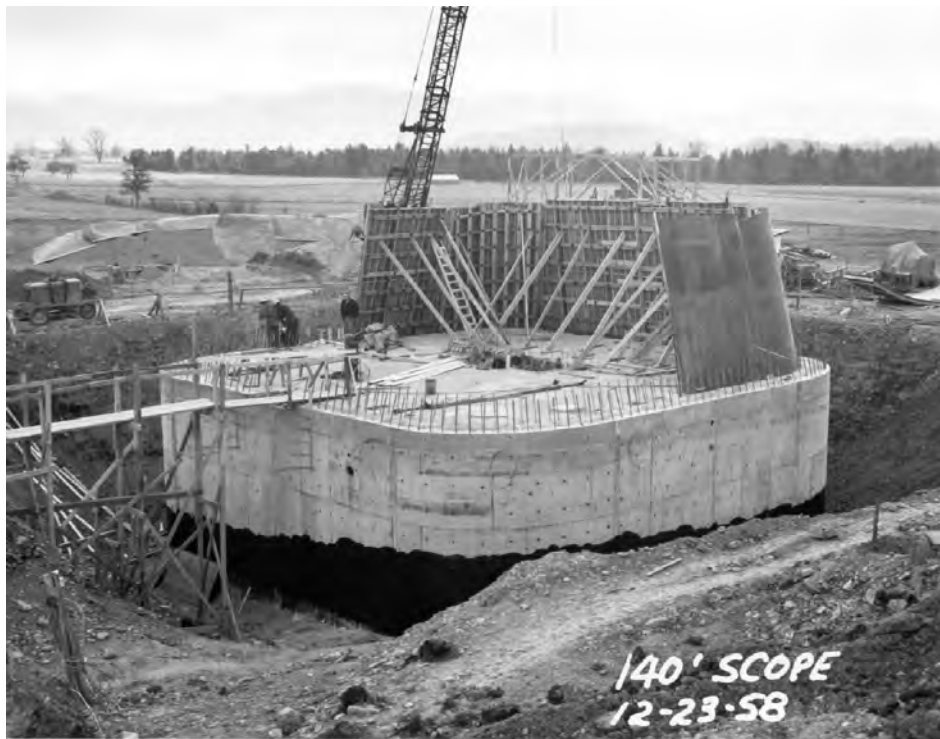
The foundation of the 140 Foot Telescope.
