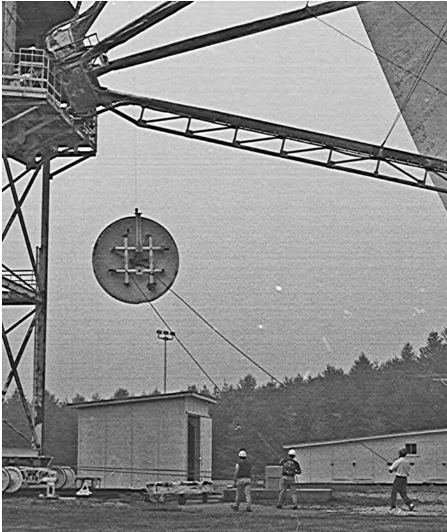
The subreflector of the 140 Foot being removed for the last time, August 1999.
