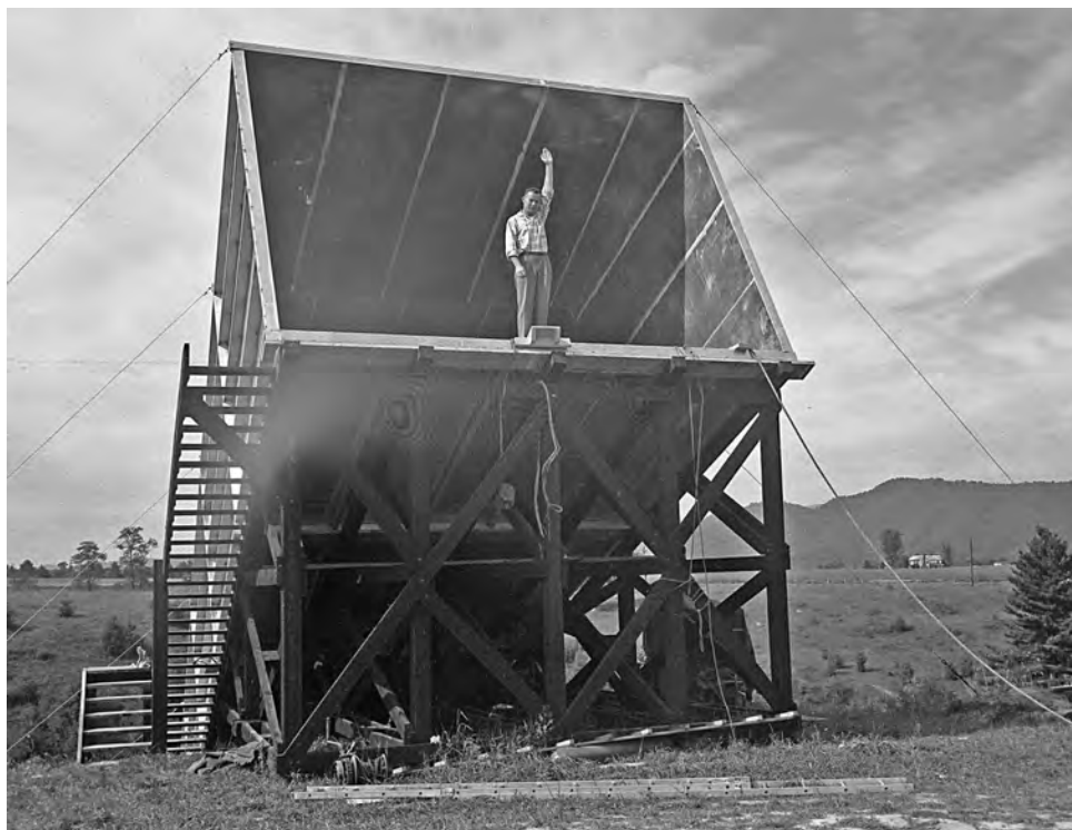
Warren Wooddell in the completed Horn.
