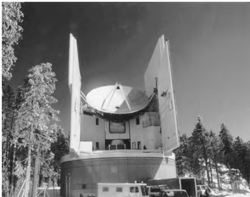
Fig. 5— The Submillimeter Telescope (also known as Heinrich Hertz Telescope, HHT) at 3200 m altitude on Mount Graham, Eastern Arizona. The 10 m diameter reflector and its backup structure employ extensively carbon-fiber reinforced plastic, which makes the telescope very insensitive to thermal gradients. Its performance during the day under illumination by the Sun is not noticeably impaired. The surface accuracy, measured and set by use of satellite holography at 37 GHz, is 20\mu at present (fall 1995) and will be improved to better than 15\mu in 1996. The Submillimeter Telescope Observatory is a joint effort of the Max-Planck-Institut für Radioastronomie, Bonn, and the Steward Observatory of the University of Arizona, Tucson.
