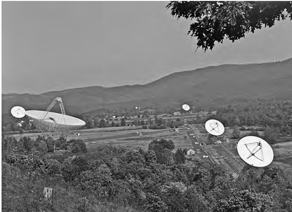
Fig. 5— The Three-Element Interferometer. This scene from 1971 shows the three elements, the Control Building, and the relay tower used to transmit and receive signals to and from the remote antenna.
