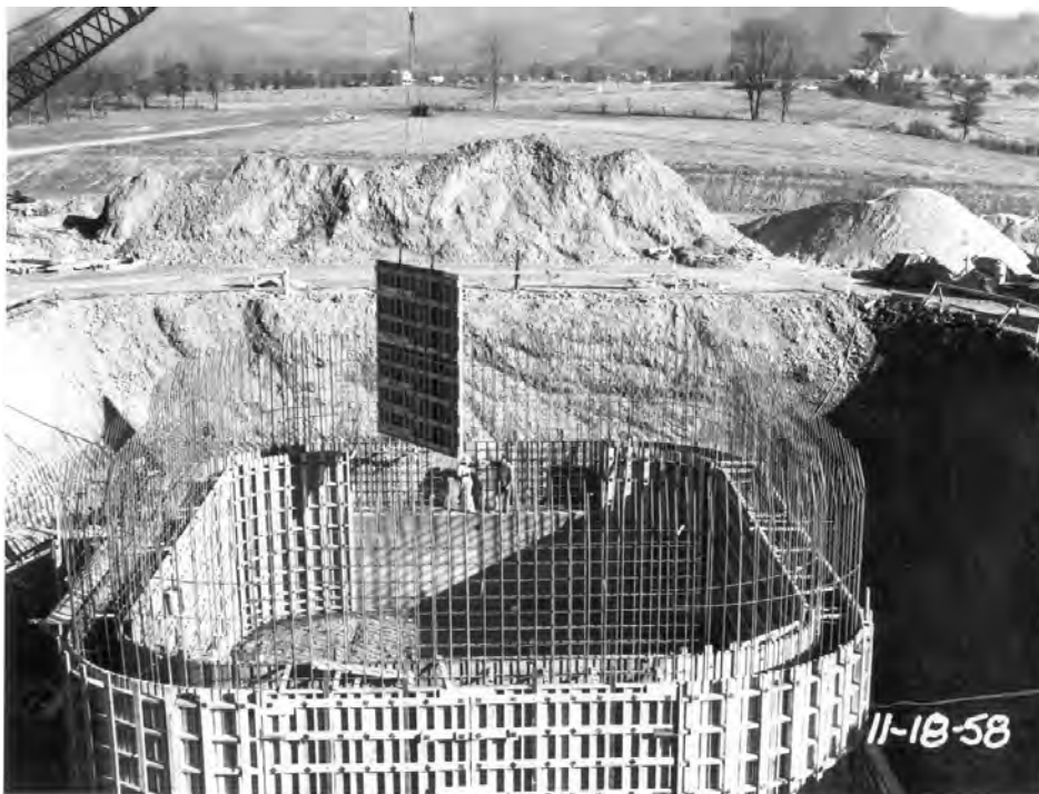
The foundation of the 140 Foot telescope under construction in November 1958.
