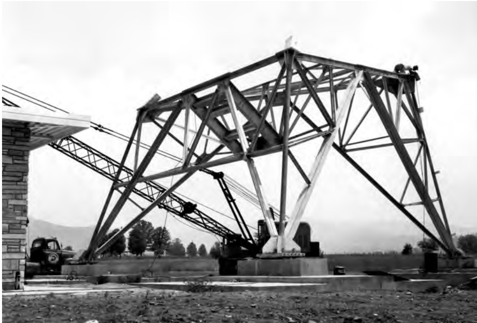
The base of the 85 Foot Telescope under construction, August 1958.
