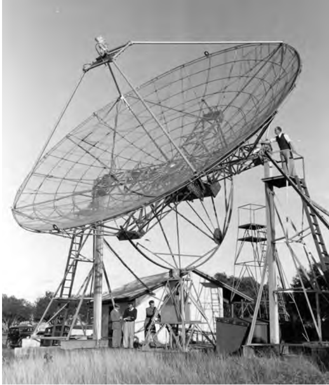
Fig 1. — The 36 Foot transit telescope at Potts Hill, near Sydney, used for early 21 cm work.
