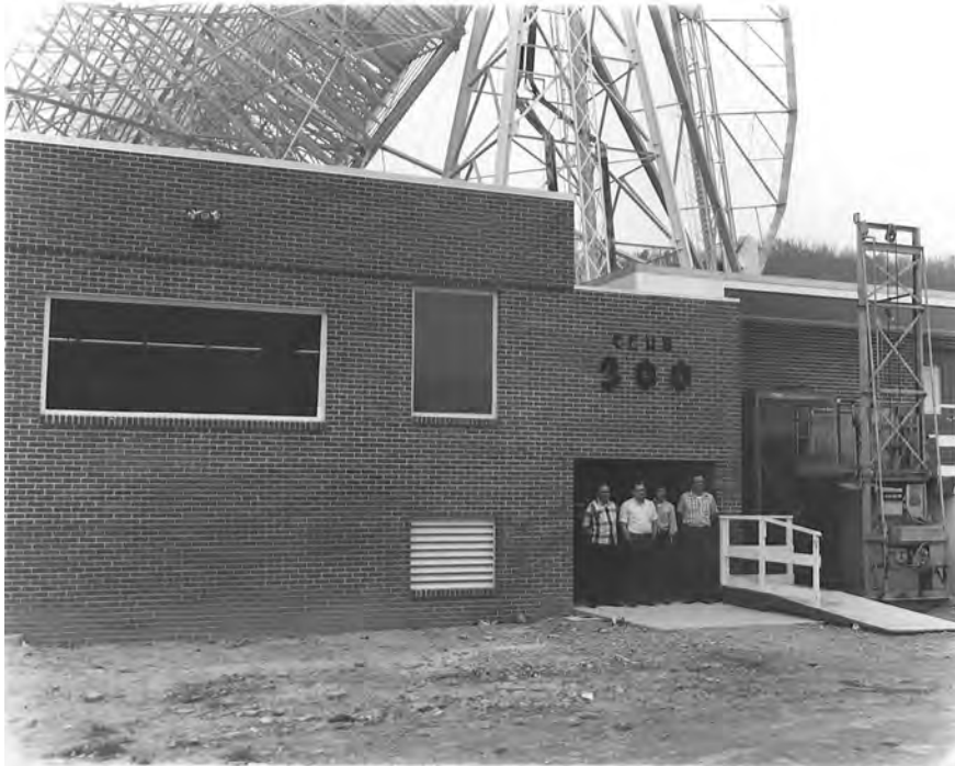
The new 300 Foot Telescope control building addition in November 1971. Left to right: Bob Viers, Troy Henderson, George Liptak, Al Hogan.
