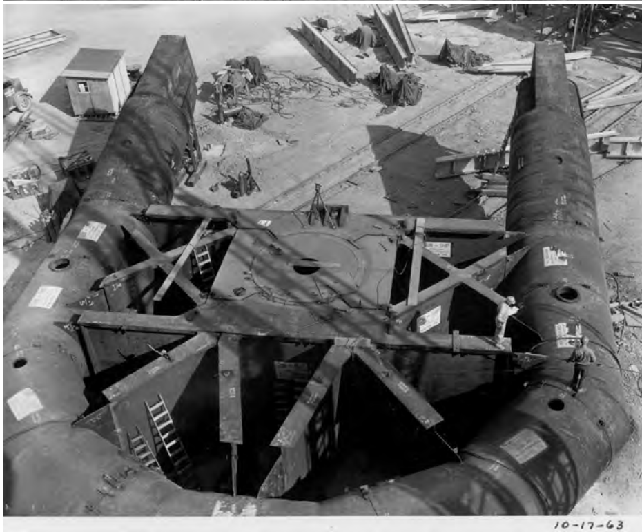
Top: The aluminum backup structure in 1962. Behind it can be seen the Calibration Horn, the 40 Foot Telescope and the 85 Foot Tatel Telescope. Bottom: The yoke being assembled on the ground, October 1963.
