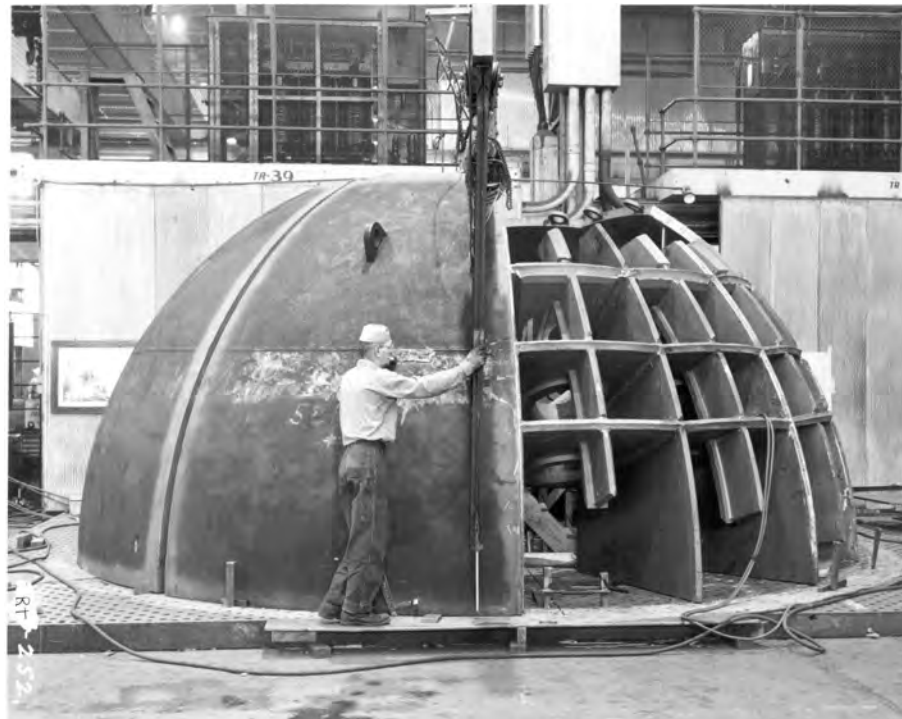
Early stages of fabrication of the Ashton-design 22 foot diameter welded spherical bearing at E. W. Bliss. [Bliss photos courtesy M. Popovich]
