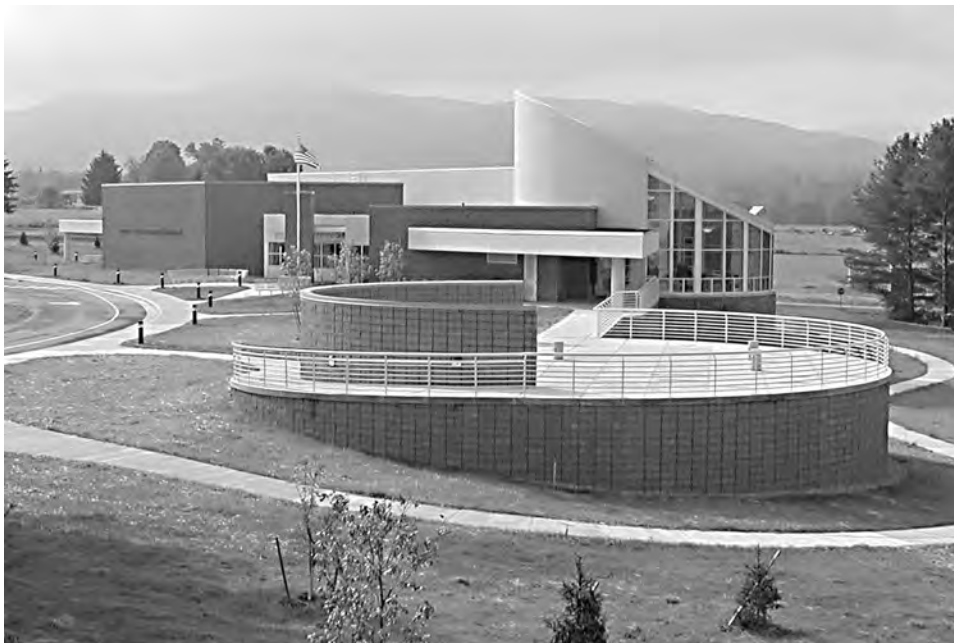
The new Green Bank Science Center, opened in the Spring of 2003.
