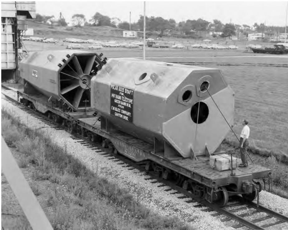
The two parts of the first 140 Foot polar shaft, loaded at the E. W. Bliss Company for shipment to Green Bank. [Bliss photo courtesy M. Popovich]
