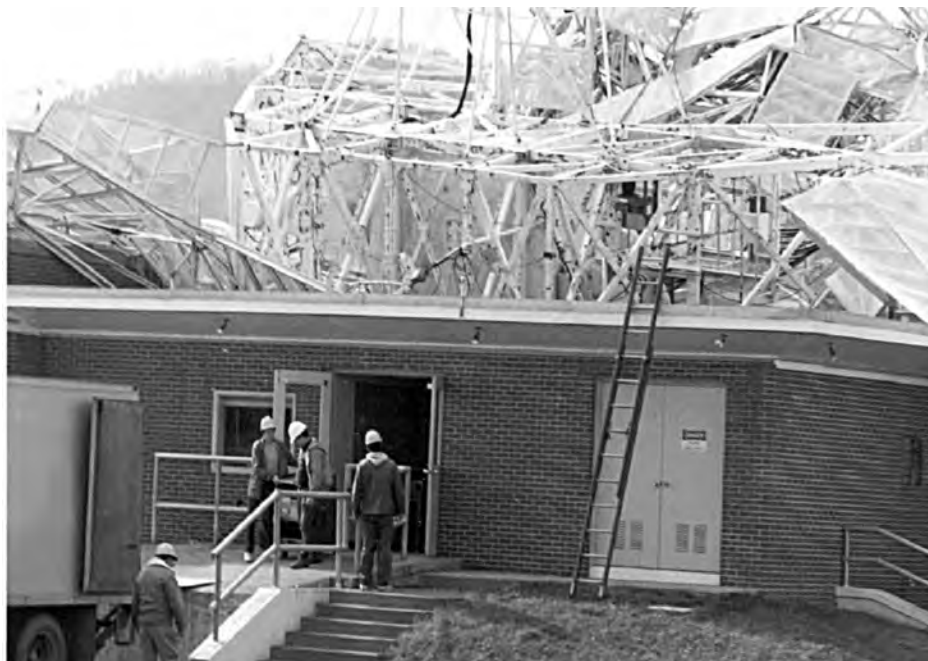
The control building.
