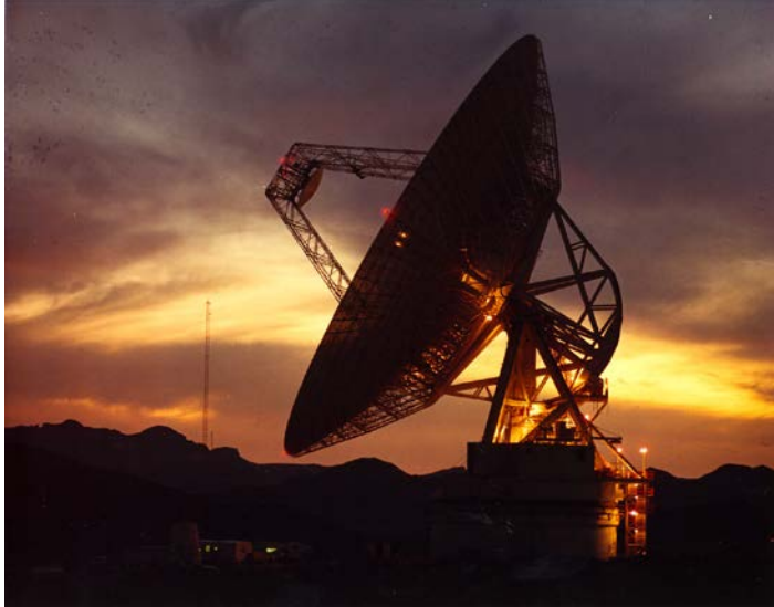
Goldstone DSS-14 (DSN) 70 m antenna, 500 kW transmitter, 4 cm wavelength (X band)
