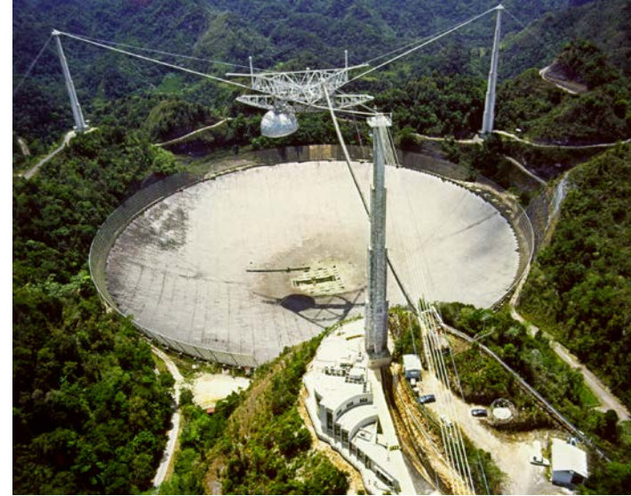
Arecibo (NAIC) 300 m antenna, 1 MW transmitter, \lambda 13 cm (S band)
