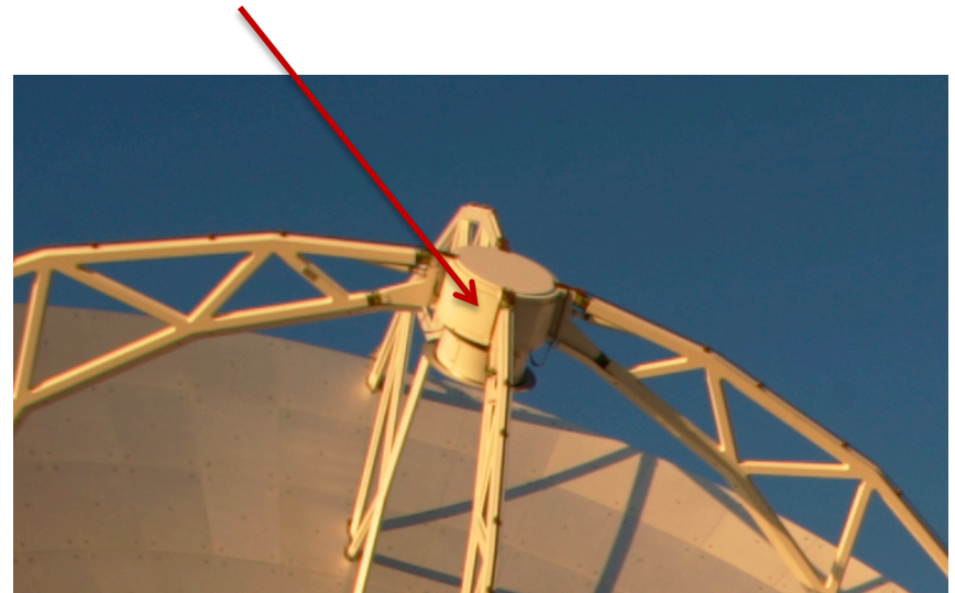
S/R Positioner support structure
