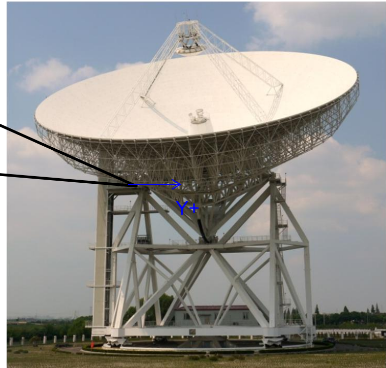
Fig. The antenna structure of TM65m on the right; a zoom of the inclinometer located on the upper part of the alidade on the left.
